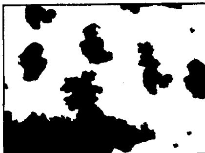
Rust Grade 2-G 33% Rusted
